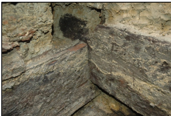
Fig. 6. Lining with cross halving joints.
