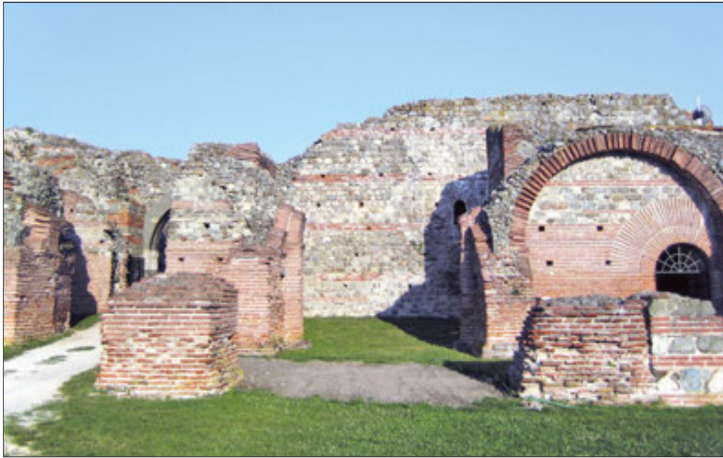
FIGURE 28. Porta decumana of earlier fortification
