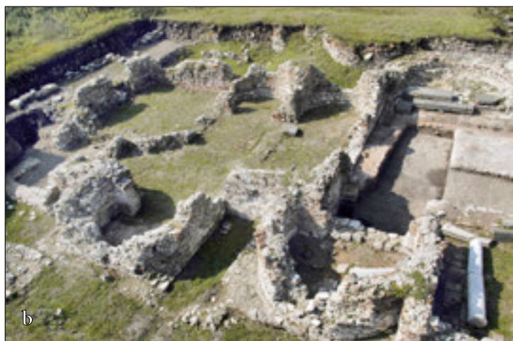
FIGURE 144. Plan of Galerius' thermae (a) and situation in 2002, before conservation and restoration works (b)
