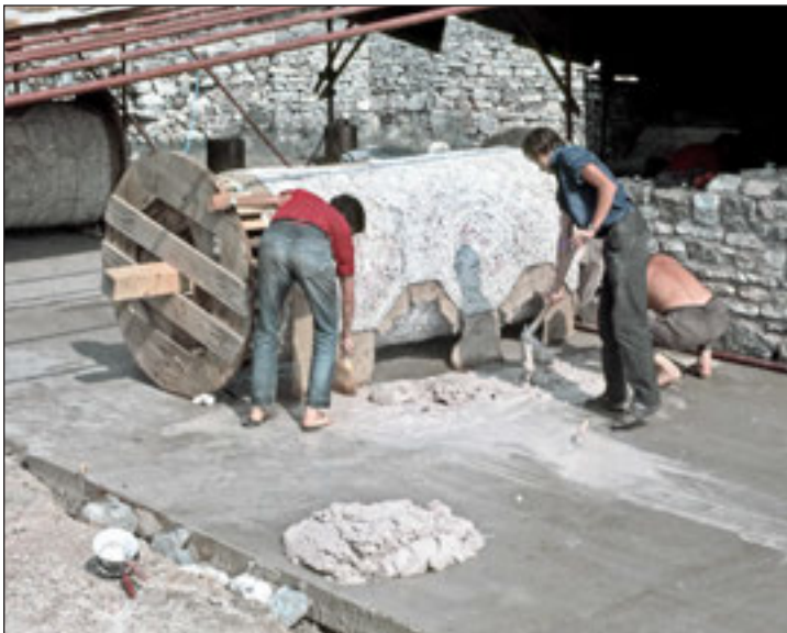
FIGURE 9. Removing of mosaics from the palace floors in 1960s
