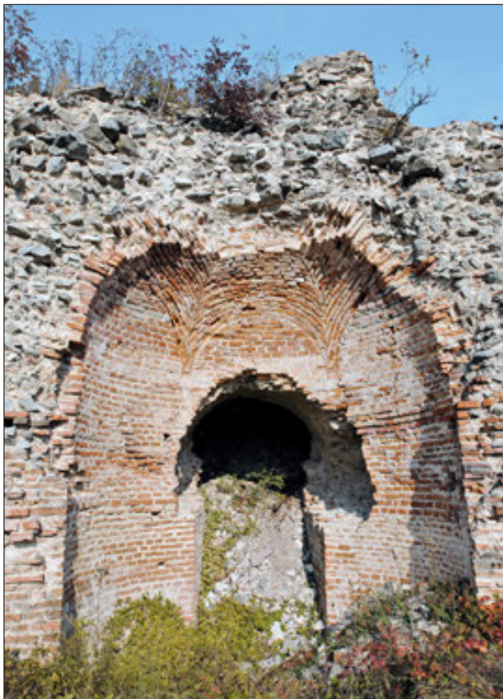
FIGURE 40. Entrance to the corner tower 15 of later fortification
