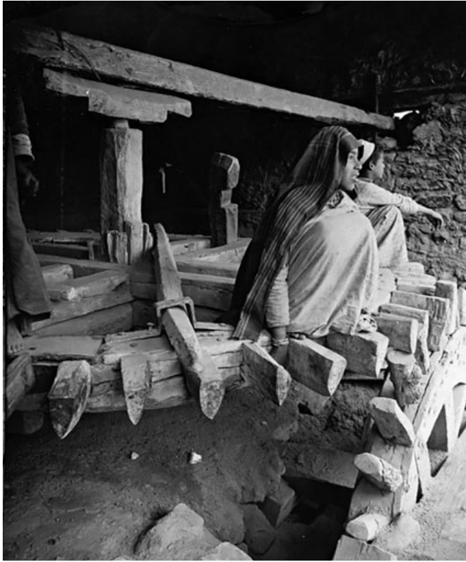
Fig. 52. Horizontal wheel of a sakīya at Saladin's Well ( Bir Yusuf ) in the Cairo Citadel (University of California, Keystone Collection; UC Riverside, California Museum of Photography, https://calisphere.org/item/ark:/13030/kt8489r2bo/ )
