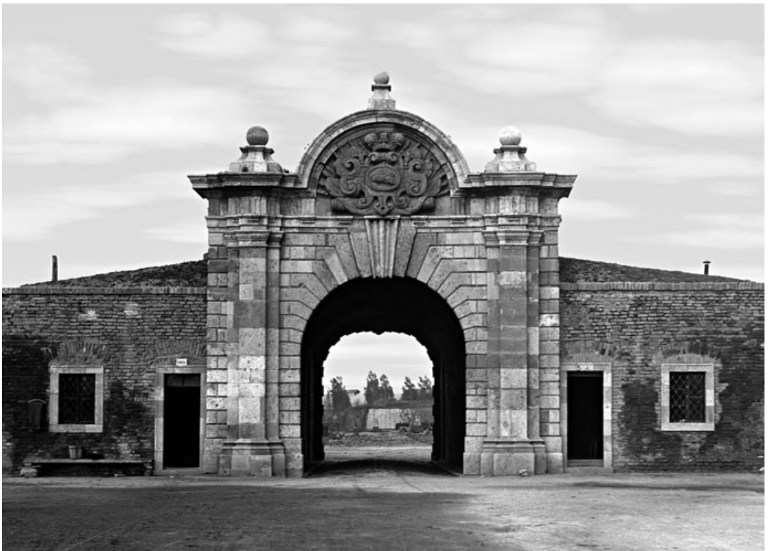
Fig. 20. Gate of Charles VI in the Lower Town, 1942 photo (Documentation of Belgrade City Institute for the Protection of Cultural Monuments)
