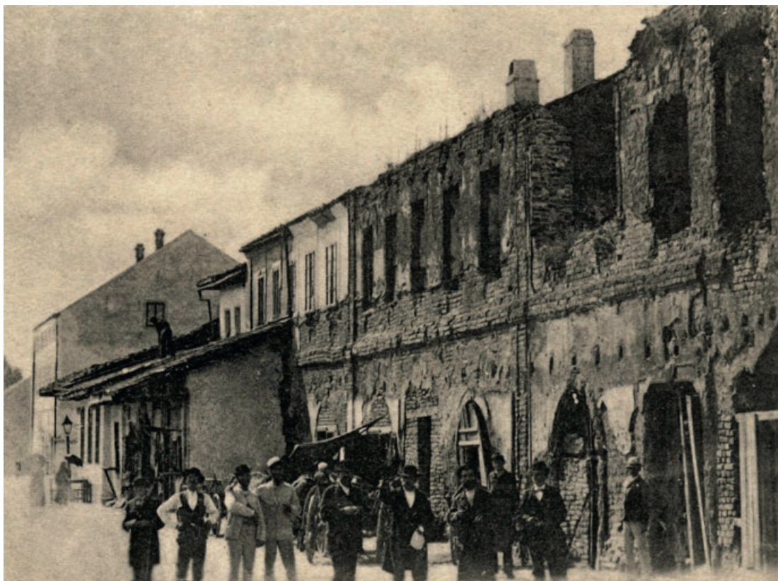
Fig. 68. View of a row of houses in Cara Dušana Street in the early 20 th century (photo archives of Miloš Jurišić)
