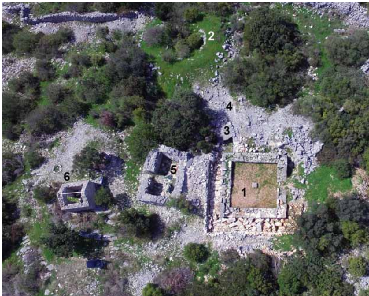
Fig. 2. Aerial view of the tower at Maslinovik and surrounding buildings made during excavations in 2017. 1. Tower, 2. Lime kiln, 3. Small drystone hut, 4. Drystone ramp. 5. Drystone house, 6. Station. Photo by E. Visković (numbers by B. Kirigin).
