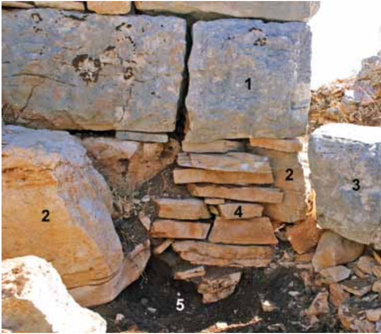
Fig. 25. The south-western corner seen from the west. 1. The corner block with drafted edge. 2. Bedrock. 3. Dislocated tower block. 4. Stacked slab stones. 5. Dark soil with recent pottery. Photo by B. Kirigin (2020).
