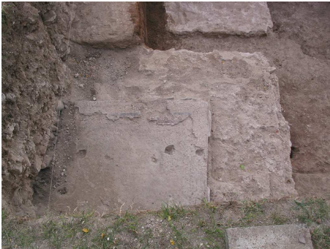
Fig. 13 Mediana, stibadium B (western triclinium), damage on mosaic (photo G. Jeremić, 2004)
