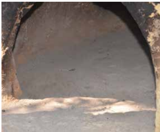
Fig. 8 – Experimental oven from 2012. after several years of usage (interior)
