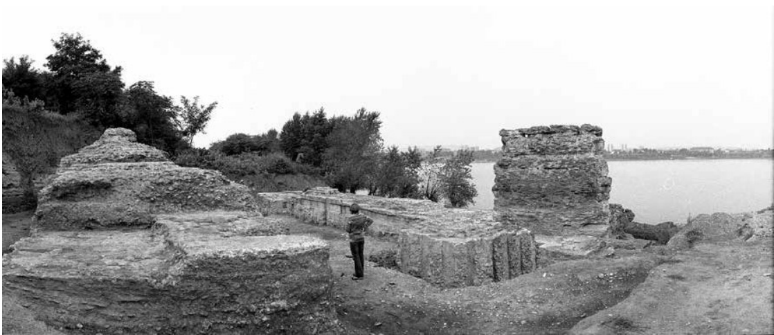
Fig. 1. The archaeological site of Pontes with the remnants of Trajan's Bridge (photo-documentation of the Institute of Archaeology, Belgrade)
