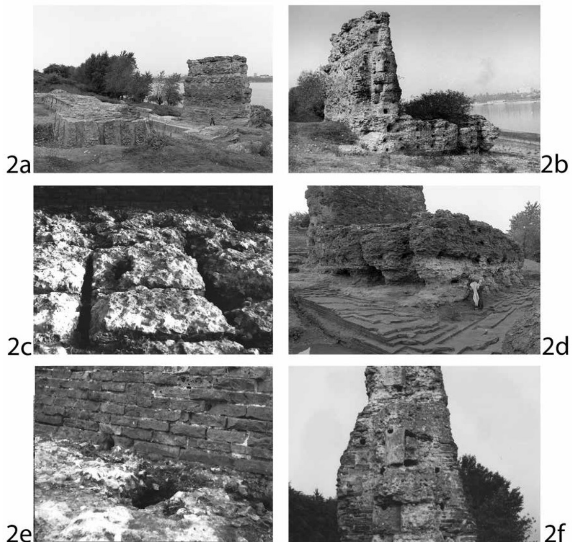
Fig. 2. a. Channels left as imprints from wooden planks of the formwork for the foundations of the first pillar in the foreground; b. The remnants of the fourth pillar of Trajan's Bridge; c. The imprints left from beams of the wooden grid system on the platform of the fourth pillar; d. Dense formation of stones and mortar tamped in the platform, with channels left from the horizontal wooden grid systems; e. a hollow left from a wooden post in the foreground of the platform and dense formation within the rows of bricks on the wall ( opus testaceum ); f. The only preserved ashlar and imprints from other missing ashlars on the side of fourth pillar; on their upper and bottom surfaces the channels left from wooden grids can be seen (photo-documentation of the Institute of Archaeology, Belgrade).
