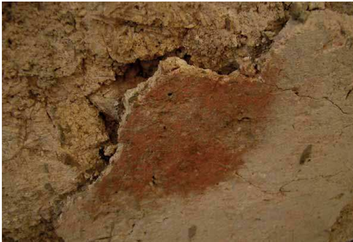
Fig. 16 Outer wall of Viminacium thermae, with red mortar having brick in its structure, detail. Photo-documentation of Institute of Archaeology Belgrade
