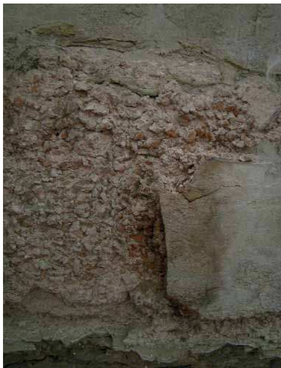
Fig. 12 Rendering layers of Viminacium thermae with brick in the form of large fragments.
