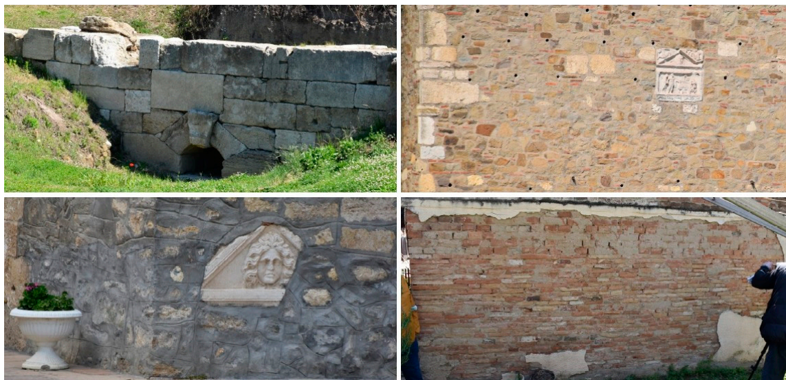
Figure 1. Stone blocks in the massive wall in Viminacium (top left); spolia assumed to be from Viminacium built in the tower of Smederevo fortress (top right); spolia assumed to be from Viminacium built in the wall of the church in Nimnik monastery (bottom left); local house wall in the village of Kostolac built of Viminacium bricks (bottom right). Photo documentation of the MoDeCo2000 project.
