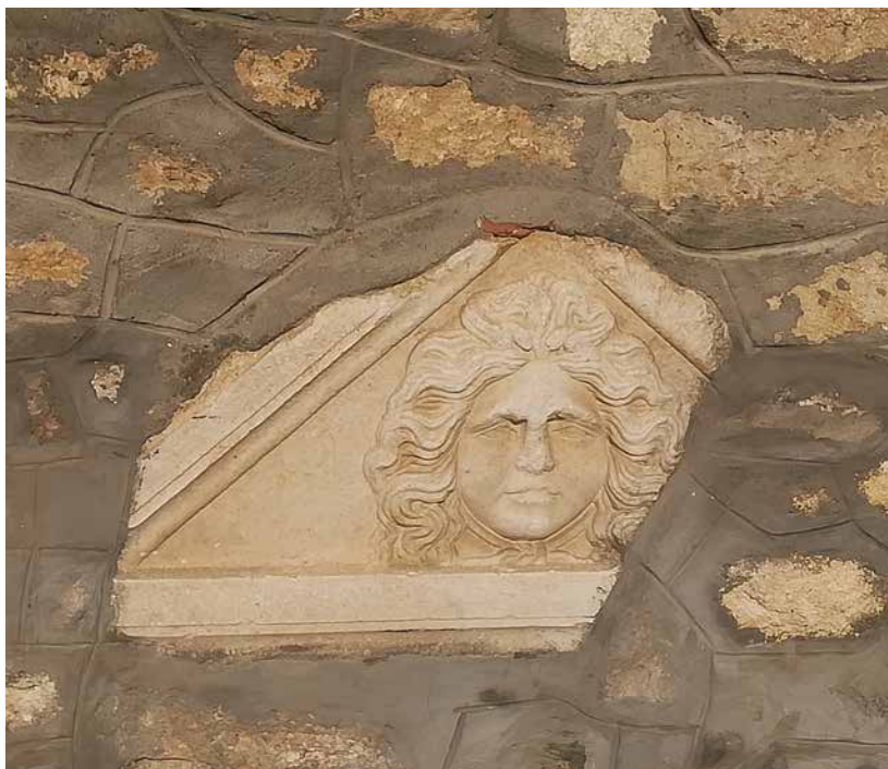
Fig. 1. Spoil built into the south wall of the Church of St. Nicholas, Nimnik Monastery (photo: Lj. Milanović)
