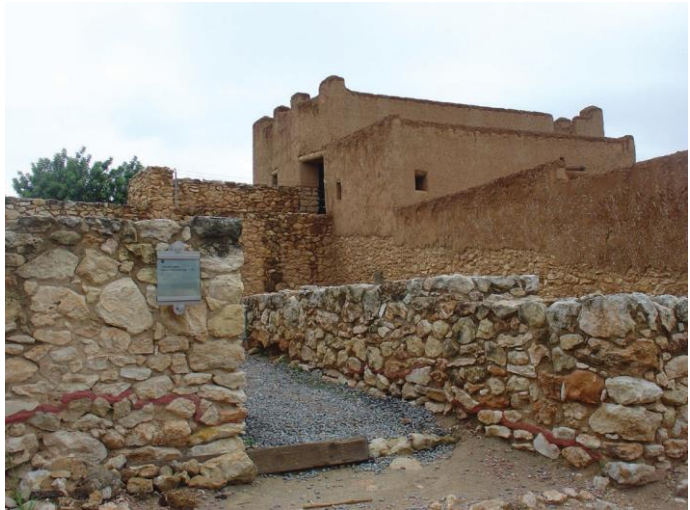
Fig. 3. Ciutadella Ibèrica de Calafell Original walls of the Ciutadella Ibèrica integrated with the reconstructed parts are separated from each other with a red strap (photo by M. Tapavički-Ilić)
