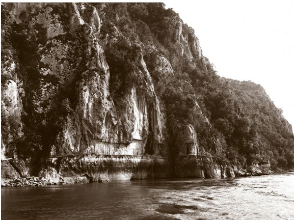
Figure 4: Roman road in the Iron Gate cut into the cliff/section at the Tabula Traiana (Photo documentation of the Institute of Archaeology, Belgrade)
