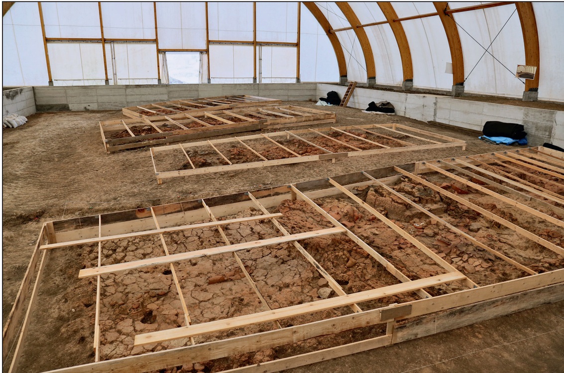
Figure 6. Added wooden construction for protection of the house remains
