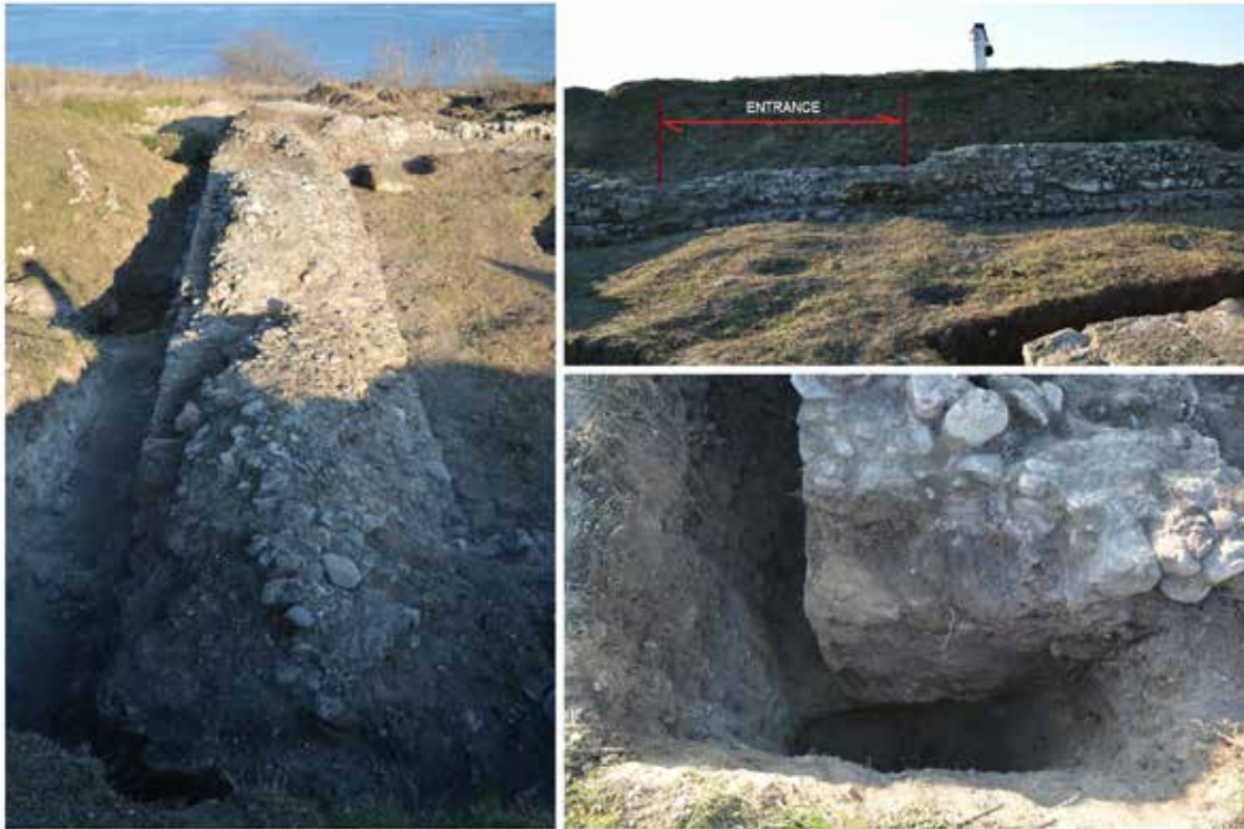
Fig. 5. Construction and masonry techniques of the foundation and above-ground zone of the rampart (photo by B. Popović)
