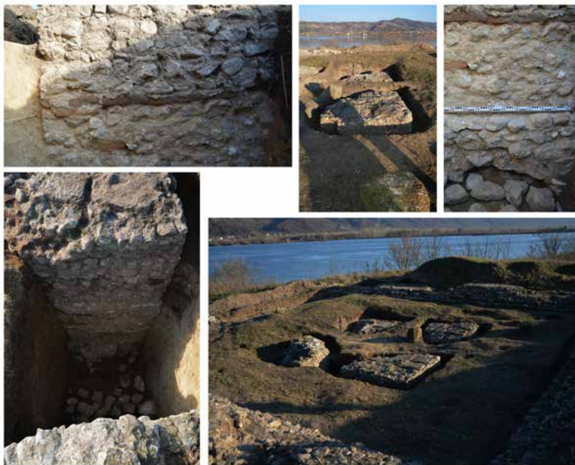
Fig. 6. Construction and masonry techniques of the foundation zone of the pillars in the interior of the fort (photo by B. Popović)
