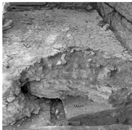
Fig. 3.2.6 : Floor in the south-eastern quarter of the P-building, seen from W (from Labraunda archive).
