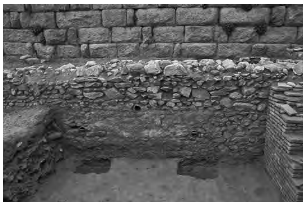
Fig. 6.4.2. : Southern face of the north wall of the roman pool (Ö. Çakmaklı).
